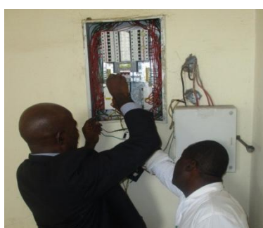
Plate 3.3.2: Installation of Logger Device on DB at REA
