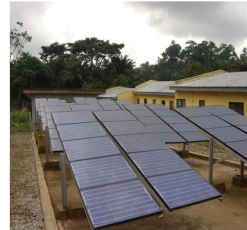
5.5 kWp Solar PV Plant at Laje in Ondo State, Nigeria.
